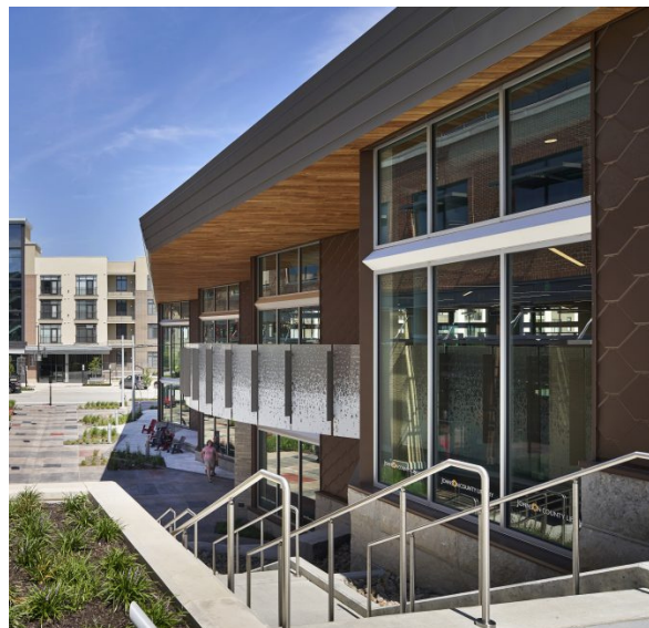
Lenexa, KS Library Black Locust Siding
